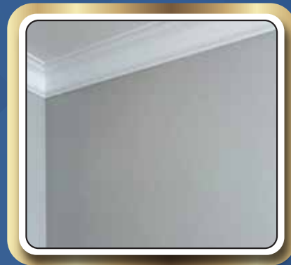
Gypsum walls insulated
